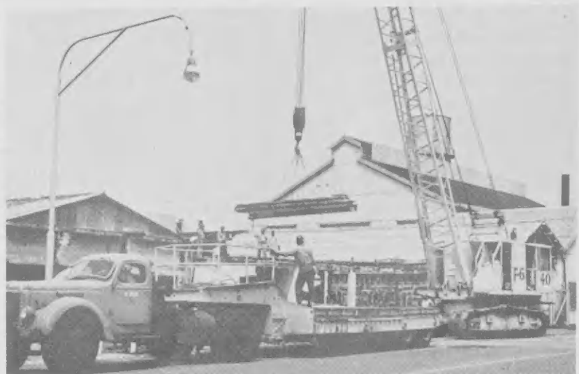
ON THIS spot, above, Lago's cold storage building stood for thirty-one years. Slabs from ceiling and walls were lifted by a mobile crane and loaded on a low-boy. They may be dumped later on the harbor reef. E LUGAR aki tabata e sitio camina e edificio di Cold Storage tabata durante trinta y un anja. Planchanan di plafond y muraya a worde lamtá cu grua y cargá ariba un "low-boy."
